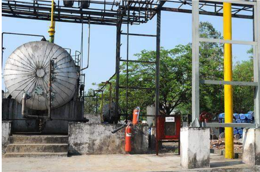
Fire Fighting Appliances Near Solvent Tank
